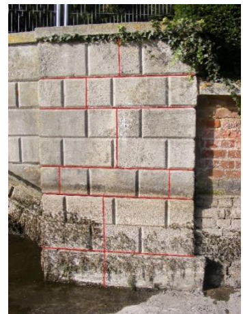
Fig 5 - the south elevation of the eastern bridge abutment, stone panels jointing.
