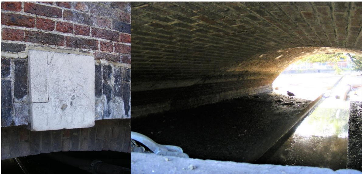
Figs 19 and 20; Lower Town Pond, North Road Bridge datestone (1828/1909) and vault soffit.
