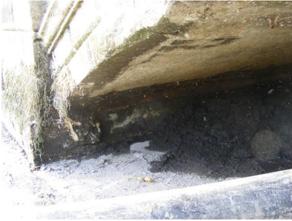
Fig 3 – the Portland stone base of the western abutment, and the springing of the brick vault.
