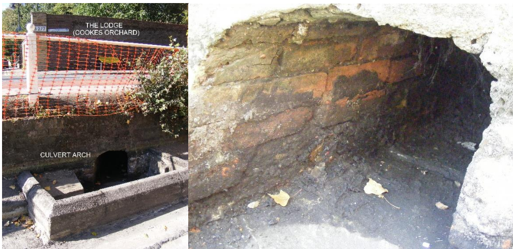
Figs 22 and 23 – Lower Town Pond, arch and culvert from the Lodge Lands
