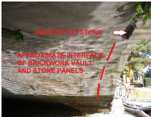
Fig 4 - the vault soffit, looking east.
