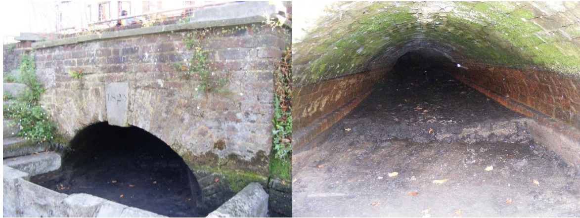
Fig 17 and 18; Lower Town Pond, south east corner, the Hog Pit arch (1823).
