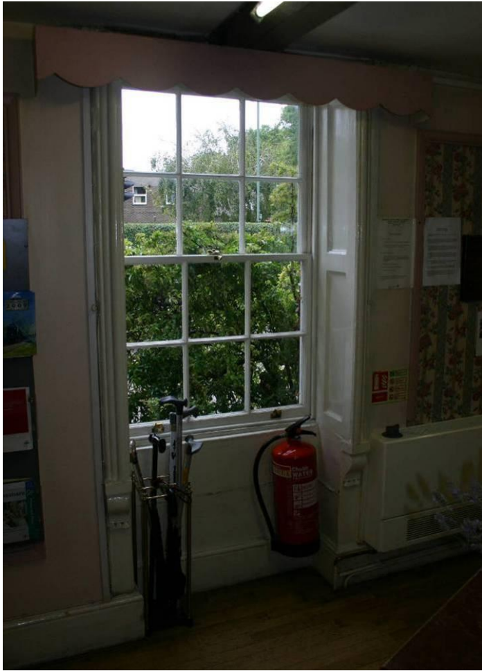
Figure 13. Front window in the central block.
