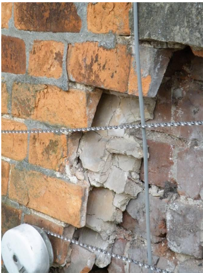
Figure 10. Detail of the mathematical tiles on the western end of the north gable of the main block.
