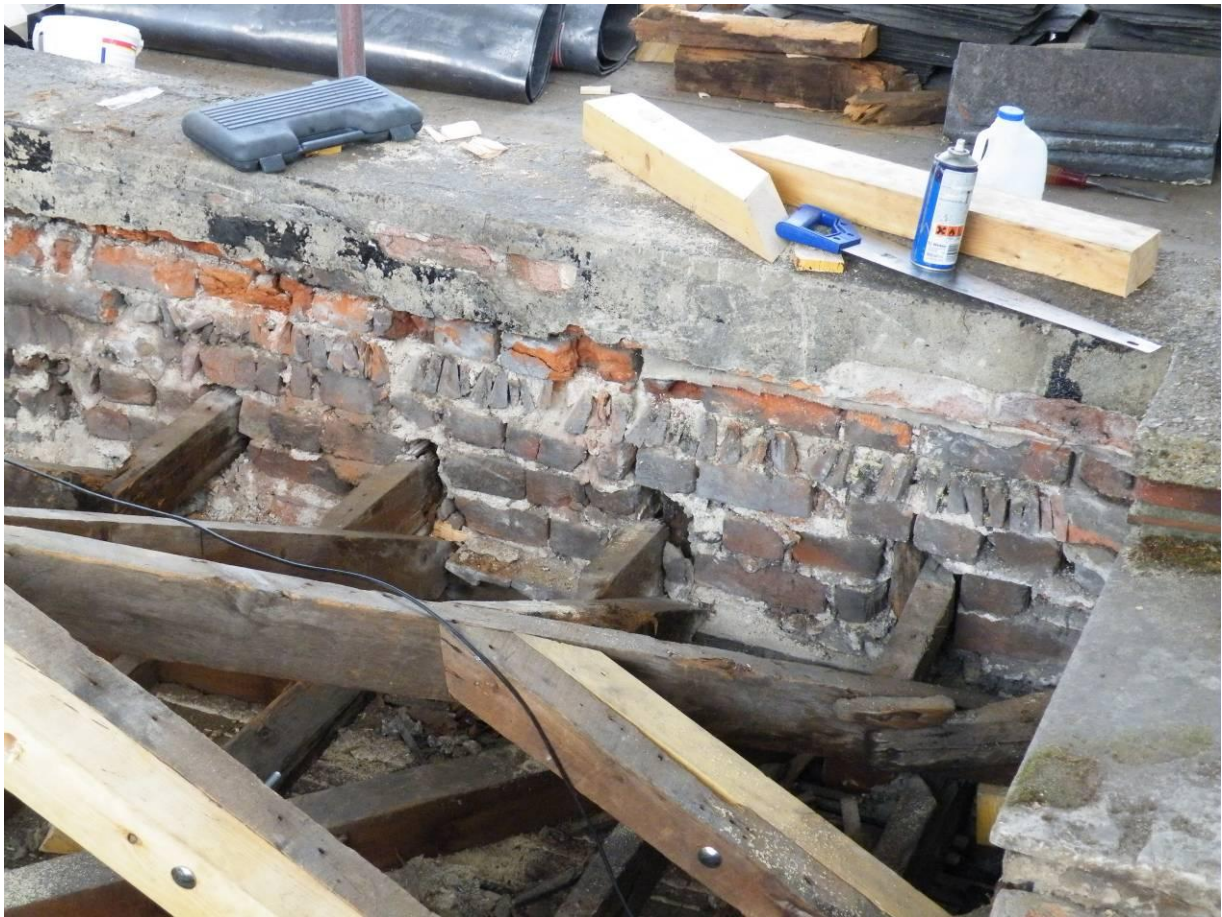
Figure 17. The wall top at southeast corner of the south extension looking east. Note the line of broken mathematical tiles.
