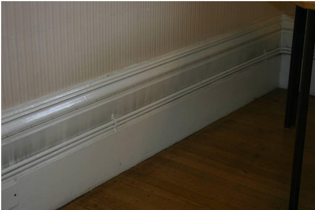
Figure 24. Detail of the skirting on south wall of the south wing.
