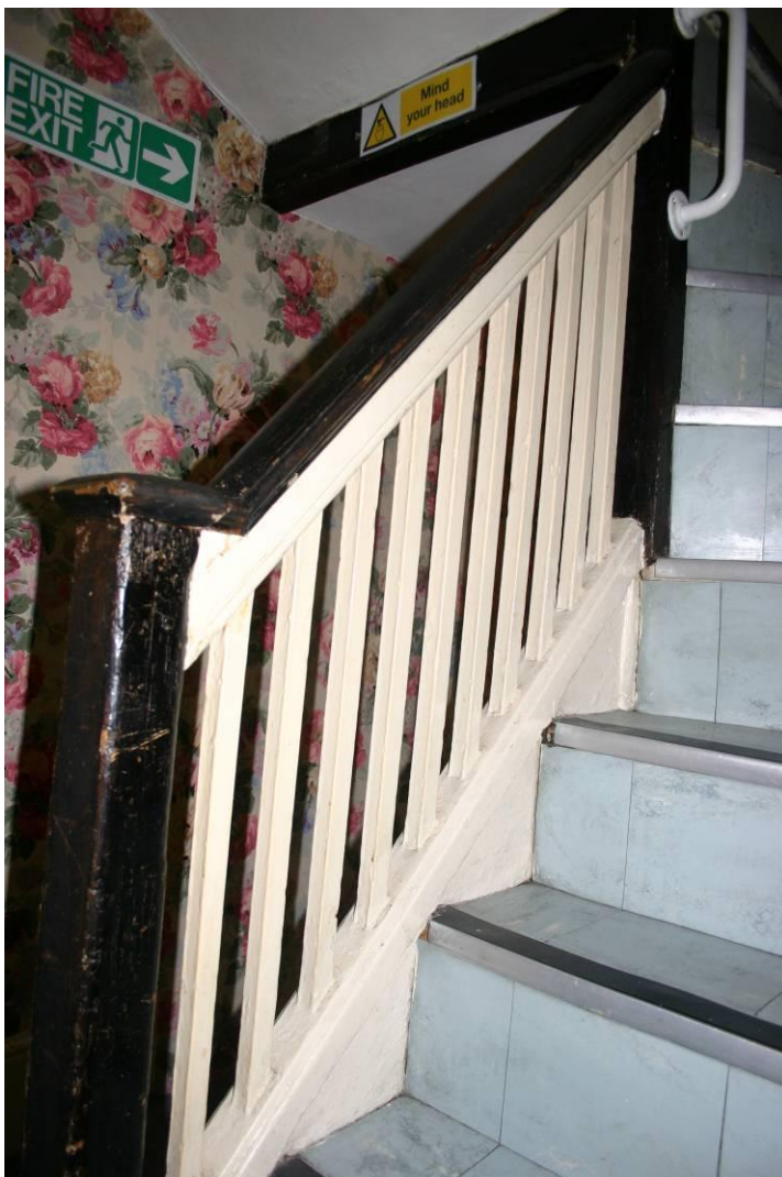
Figure 12. The staircase to the caretakers flat in the attic.
