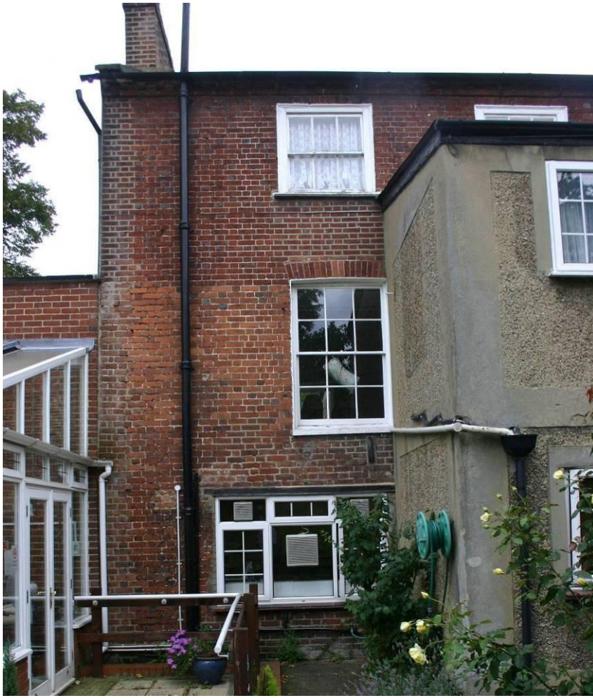
Figure 5. Central block, back, south end.
