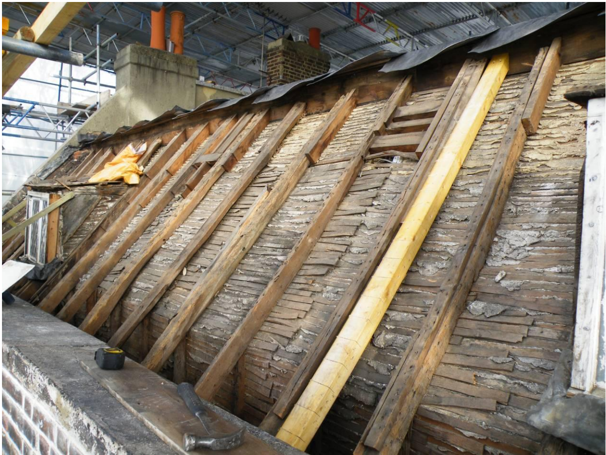
Figure 3. The front roof looking north during the repair work.
