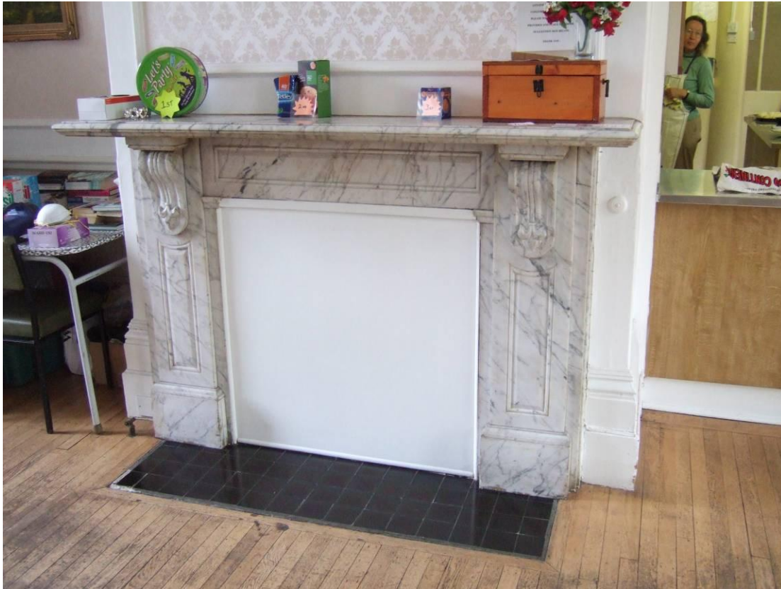
Figure 25. Fireplace in the south wing.
