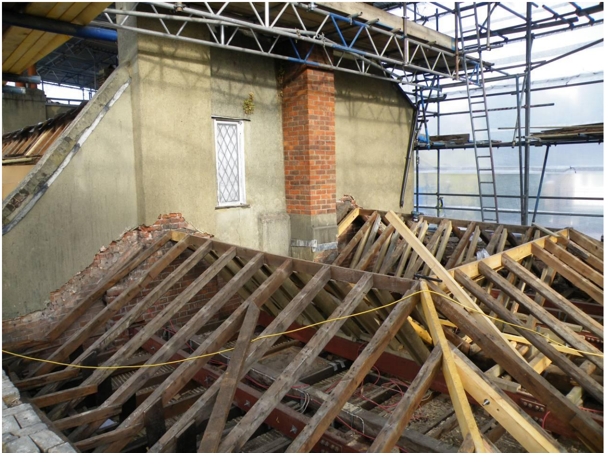
Figure 7. The south side of the main block and the roof of the south wing during building work, 3 November 2010.
