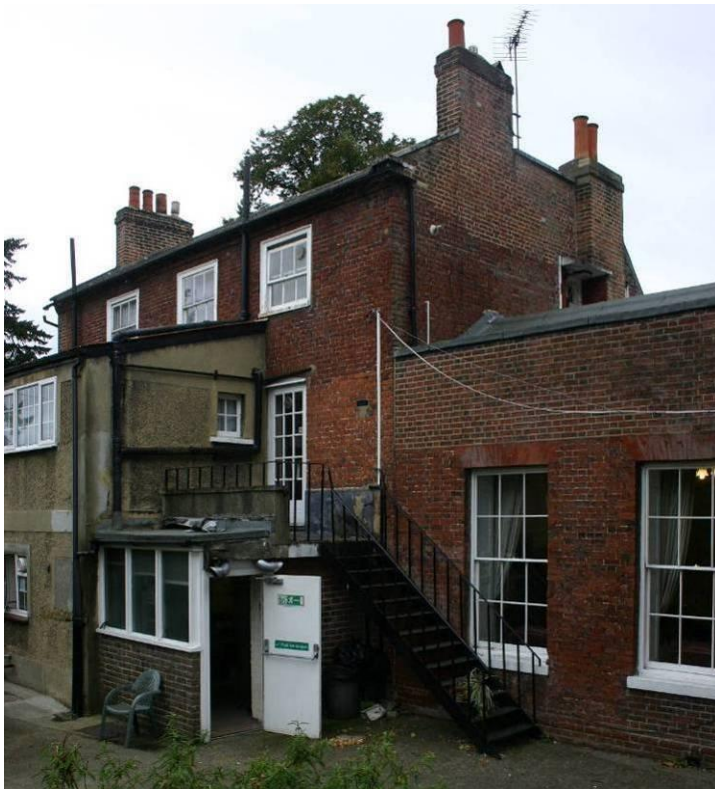
Figure 6. The back of the central block looking southwest.
