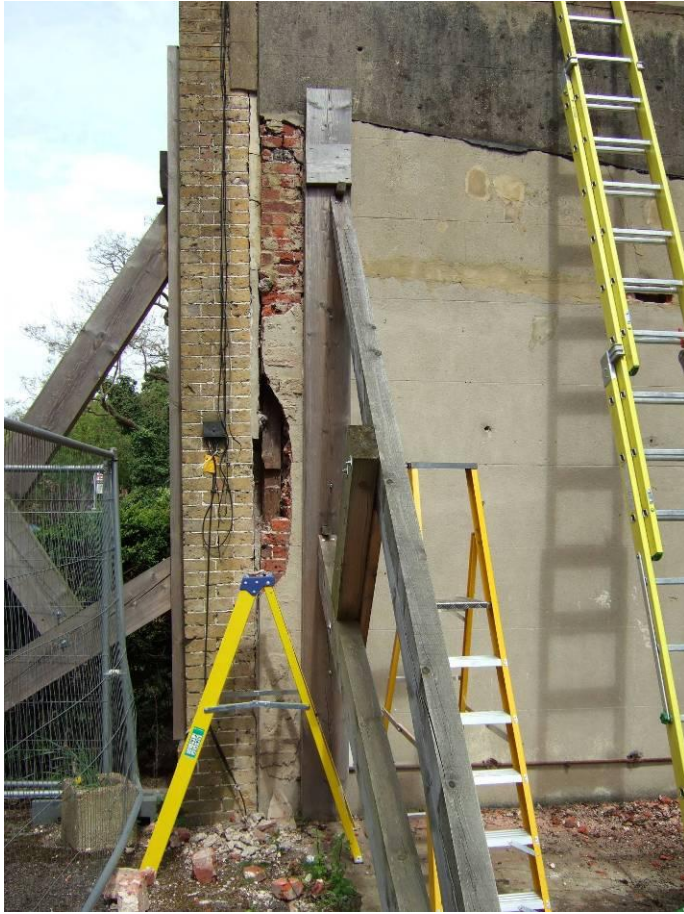
Figure 19. The western end of the south wall of the south wing.
