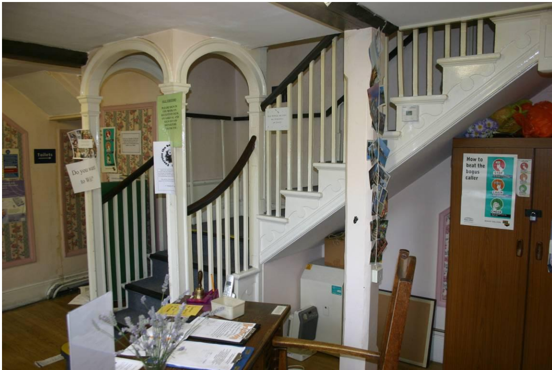
Figure 11. The staircase from the ground floor.
