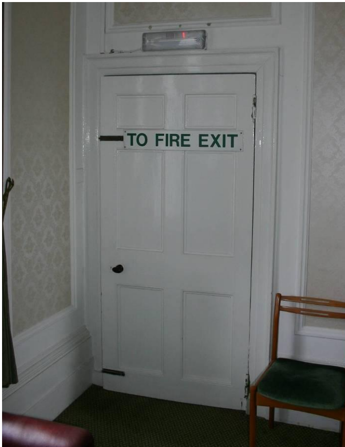
Figure 15. Door between the north wing and the central block.
