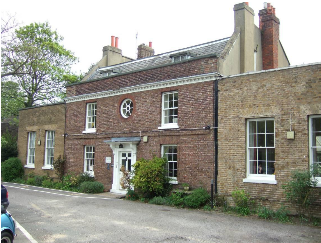
Figure 1. The front looking north.
